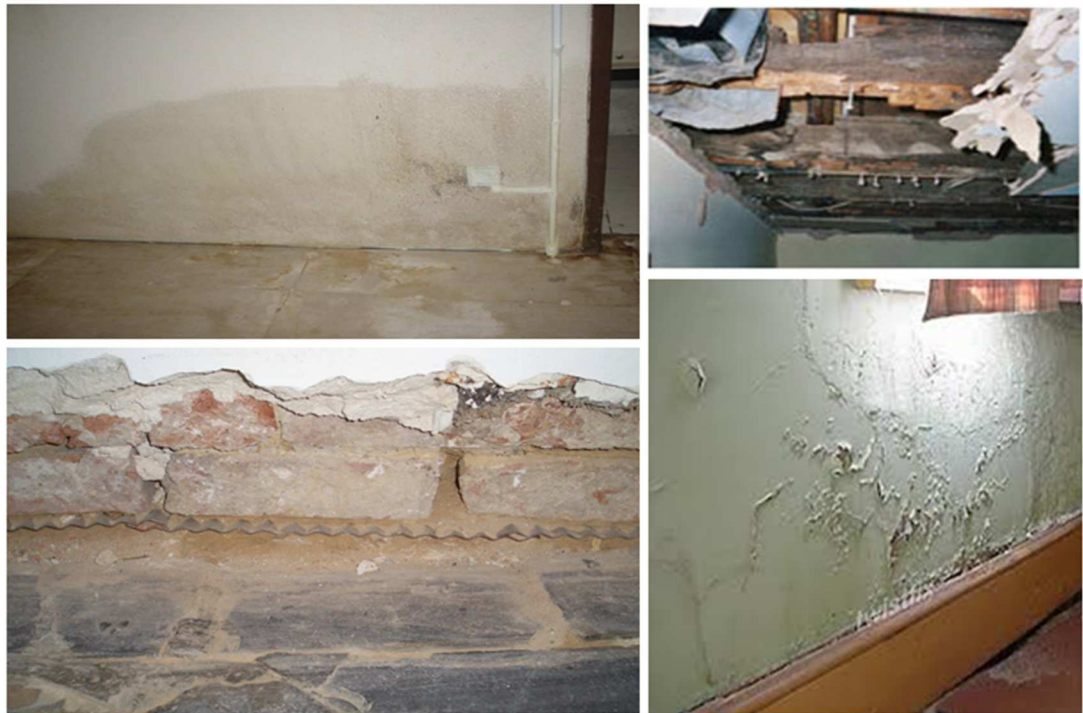
Figure (3.1) Effect of dampness
