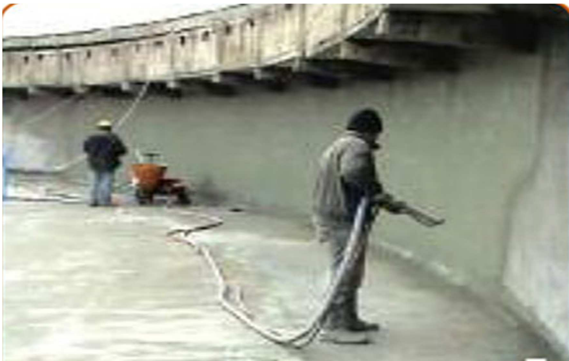
Figure (3.5) Waterproofing for a huge tank
