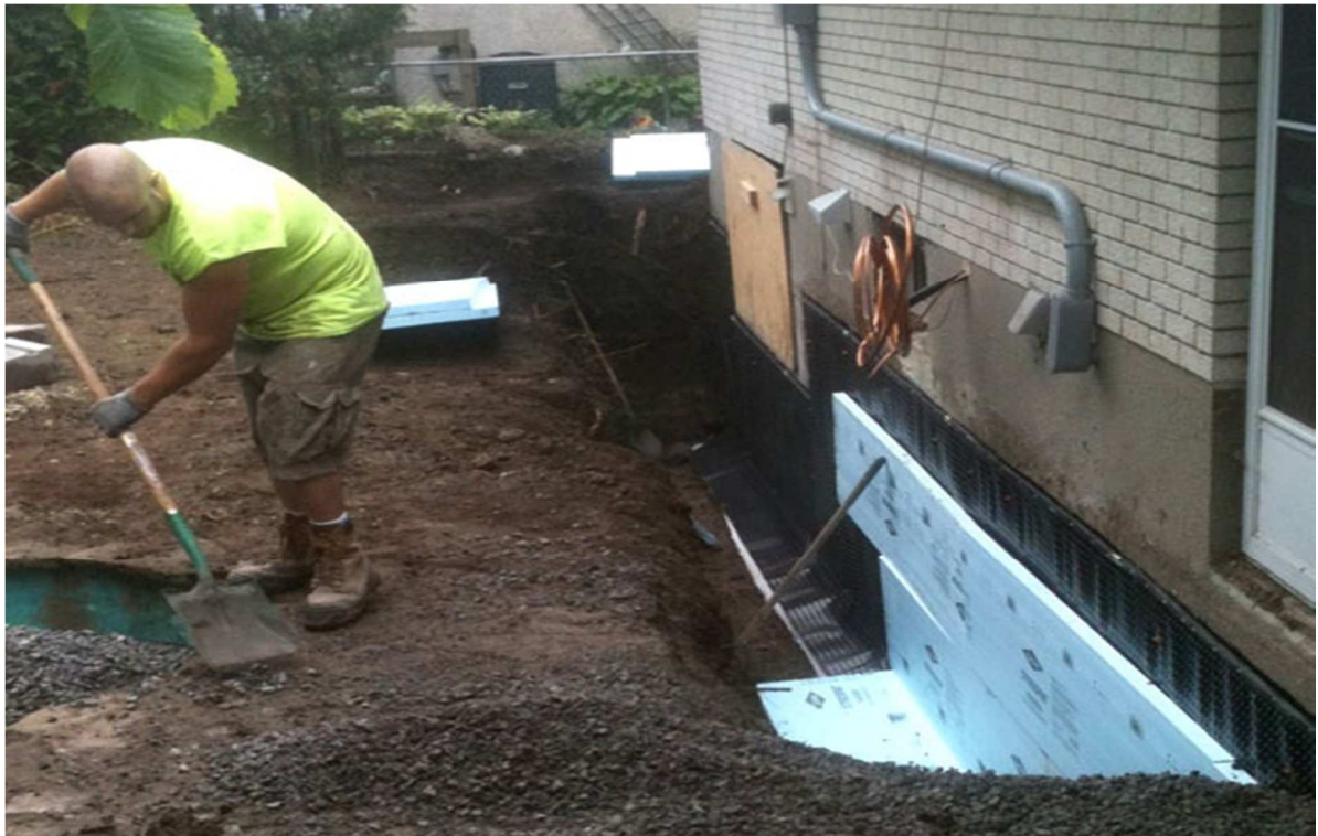
Figur (3.3) Waterproofing of foundation
