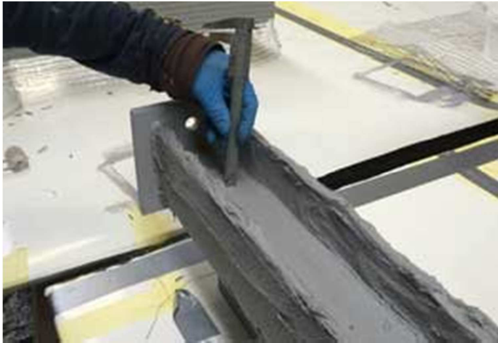
Figure (6.2) Fireproofing structural steelwork
