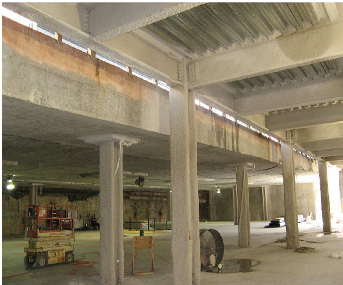
Figure (6.3) Application of fireproofing spray
