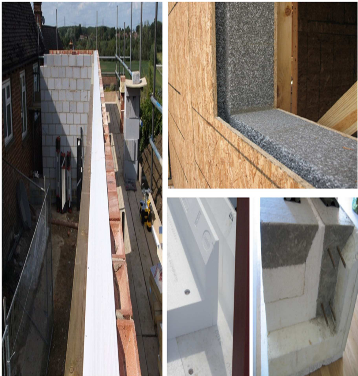
Figure (1.13) Avoiding thermal bridges
