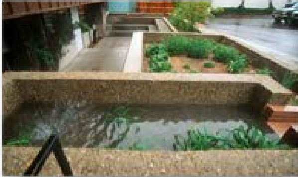
Rainwater collected in planter box then channeled into rain garden Boulder, CO
